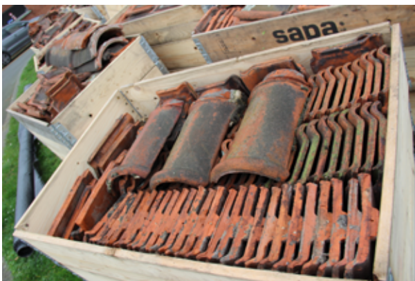
Example of storing tiles for reuse
