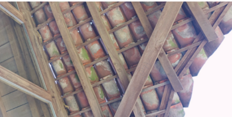
Example of the application of reclaimed roof tiles (Flemish tiles) on a 1741 building rebuilt at the KampC in Westerlo; note the reduced rainfall density of the roof due to the lower dimensional stability of the tiles; the role of the under-roof becomes very important
