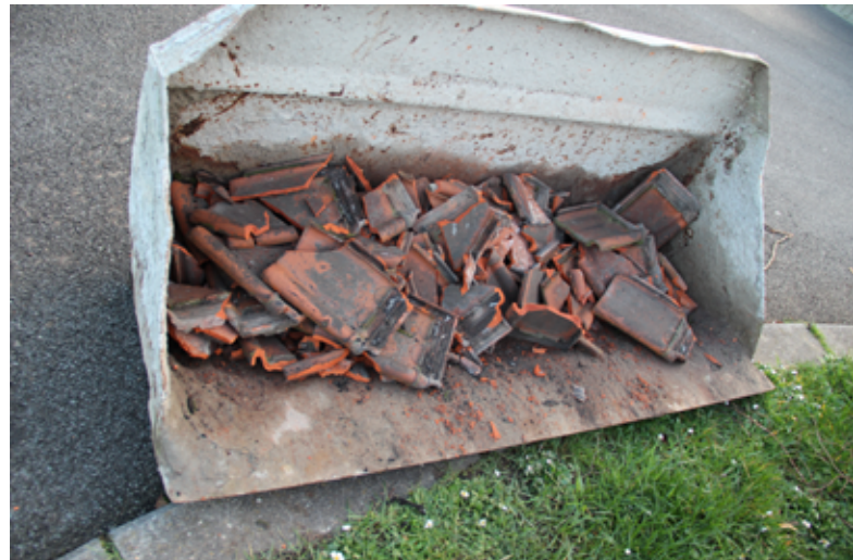
Example of sorting of remains of tiles not reusable during removal (© Buildwise, Tuighuisstraat worksite, Courtrai)
