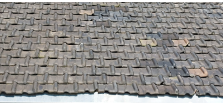
Example of the application of recycled tiles, illustrating lower dimensional stability, with an impact on aesthetics (straight lines sometimes more difficult to achieve).
