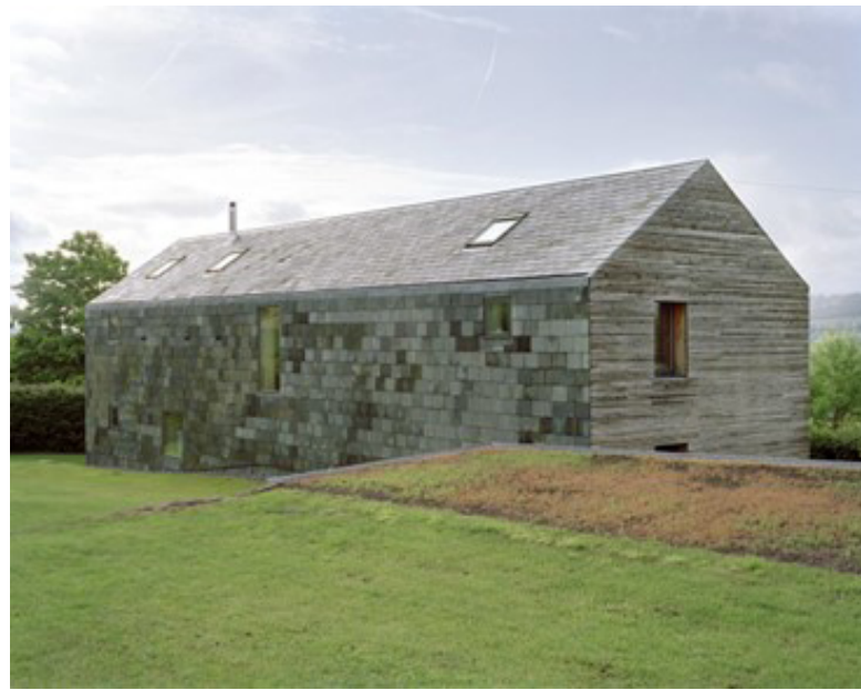
Concrete example of reuse of roofing products (natural slates): see https://opalis.eu/nl/inspiration/5599
