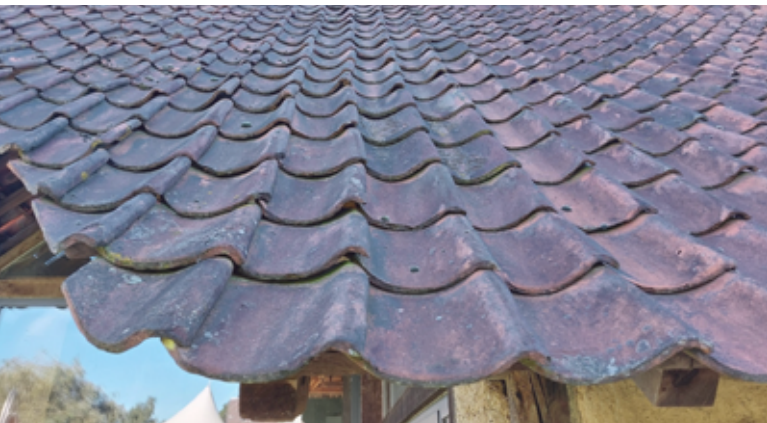
Example of the application of recycled tiles, illustrating lower dimensional stability, with an impact on aesthetics (straight lines sometimes more difficult to achieve)
