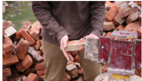
Manual and mechanical cleaning of mortar remains
