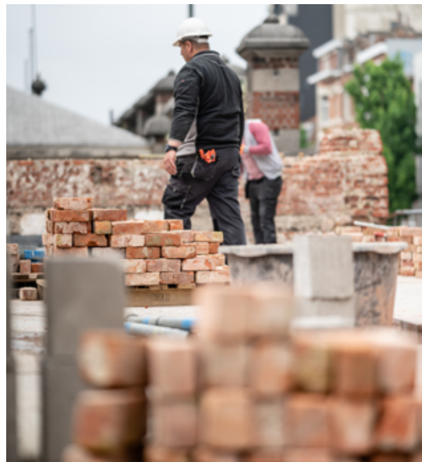
Removing bricks – Ixelles barracks © Ekkow Photography – Buildwise
