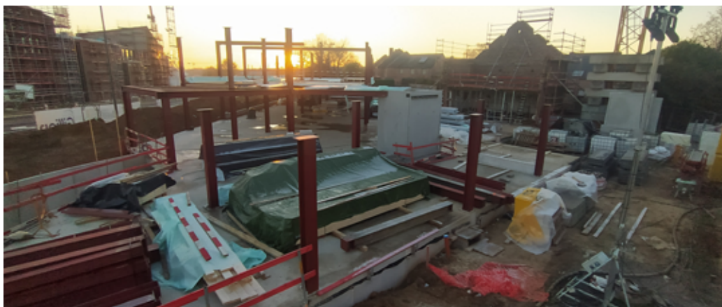
Mundo Lab worksite in Louvain-La-Neuve
