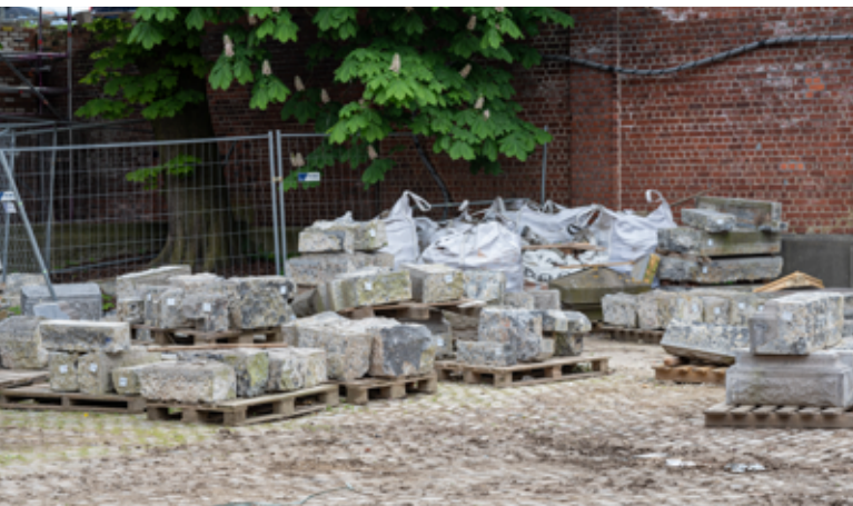
Storage of removed stone elements – Ixelles barracks
