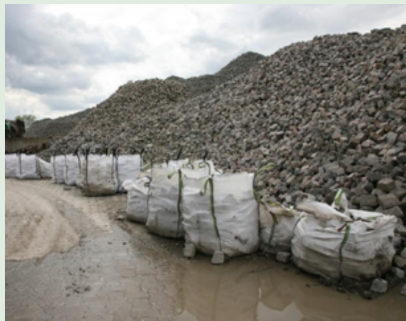
Paving block storage on site.
