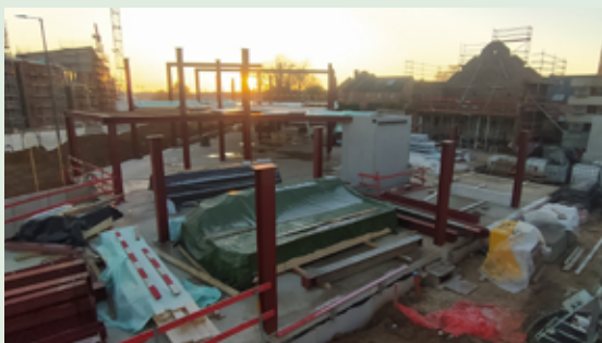
Chantier Mundo Lab in Louvain-La-Neuve, Belgium
