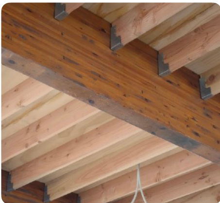
Reused glue lam beams
