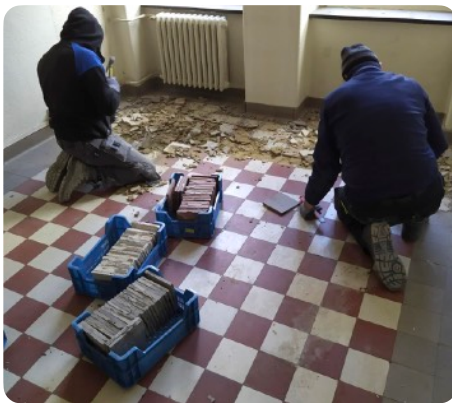
Careful dismantling of tile floor
