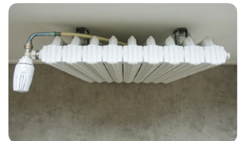
Caserne de Reuilly, Paris Habitat - In situ reuse of 85 cast iron radiators. © ROTOR and SIXIEME CONTINENT
