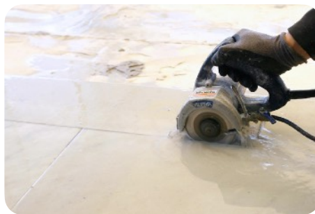
Sawing joints
