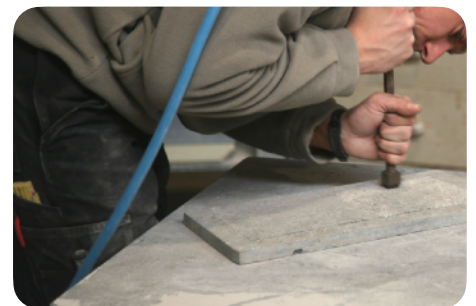
Bush hammering of slabs
