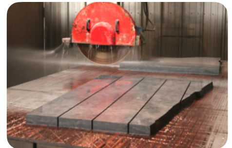
Cutting stone elements
