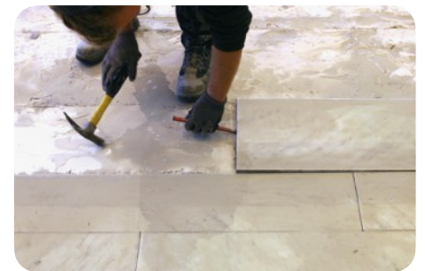
Removing the slabs
