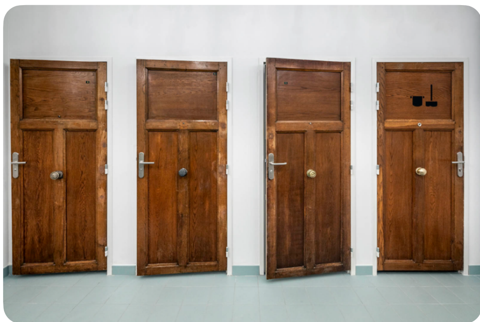
Reuse of panelled wooden doors © Cyrus Cornut, Grande Halle de Colombelles, WIP. Architects: Encore Heureux (FR)
