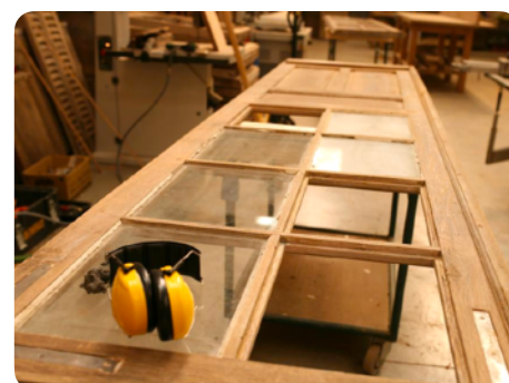
Replacement of glazing elements
