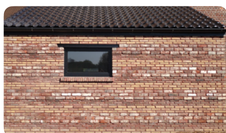
Bricklaying of a façade with three different models of reclaimed bricks. Chiro Itterbeek (BE). © ROTOR
