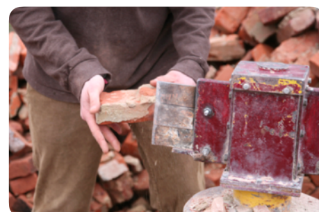
Mechanical cleaning of mortar remains
