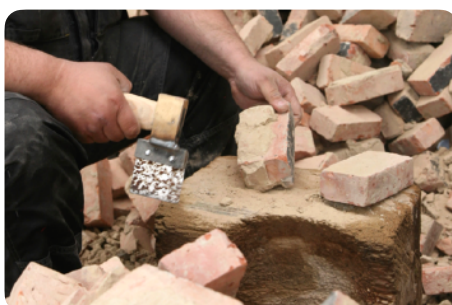
Manual cleaning of mortar remains
