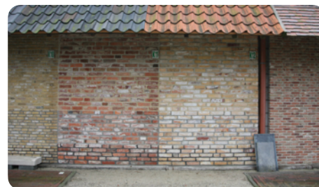
Showroom of a reseller of reclaimed bricks. Enhancement of the different models, with joints of varying nature and thickness
