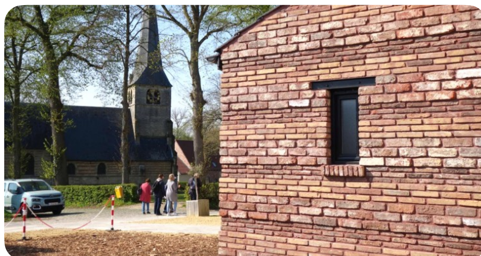
Bricklaying of a façade with three different models of reclaimed bricks. Chiro Itterbeek (BE). © ROTOR
